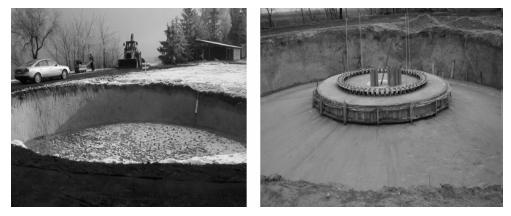
*Fig. 1* Phases of laying the foundations for the wind turbine at Kulcs (source: *www.winfo.hu*)
